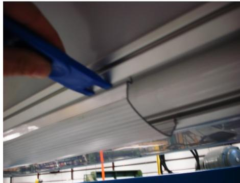
Figure 9-6, Remove Fluorescent Lens with Lamp Tube Extraction Tool
