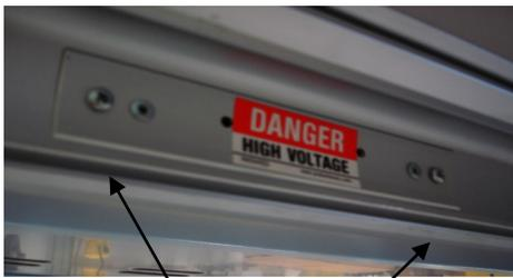
Remove Ballast Face Plate Screws
