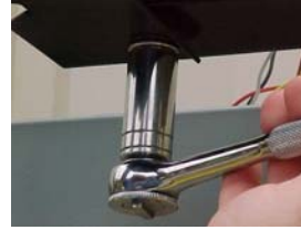
4. Remove 1/2-20 nut @ bottom of hinge w/ 3/4" wrench. Discard it.
