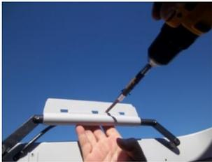
Using cordless screw gun with a #3 bit, loosen the screw on switch from the inside.
