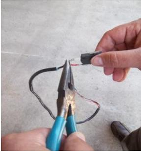
Using needle nose pliers remove top connector
