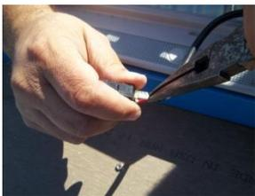
With needle nose pliers remove red and black wires from connectors
