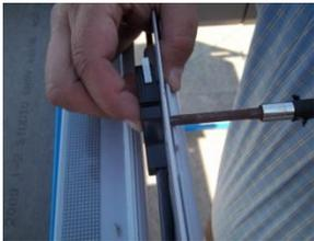
With cordless screwdriver, insert and thread ½" screw into hex nut at switch.
